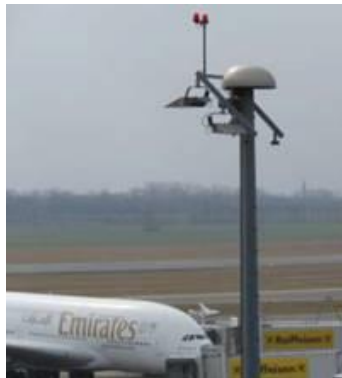
Radio installation on poles
