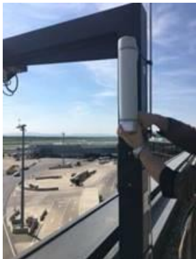
Antenna installation on rooftop
